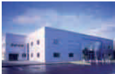
Edina manufacturing facility in Lisburn
